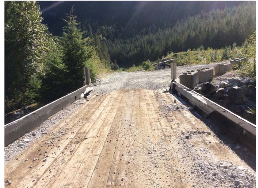
Right approach viewed from bridge
