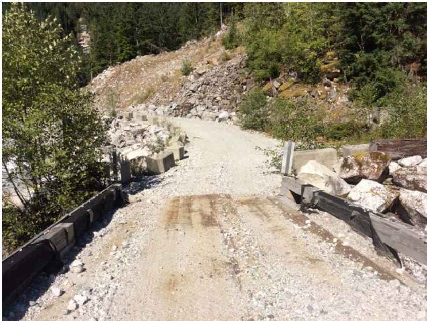
Left approach viewed from bridge
