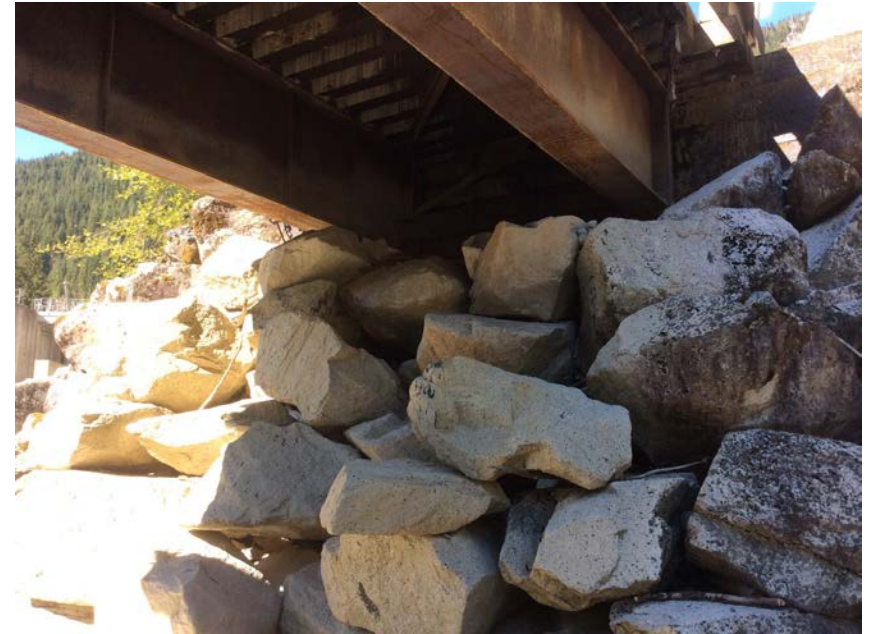
Left Bank Abutment when facing downstream
