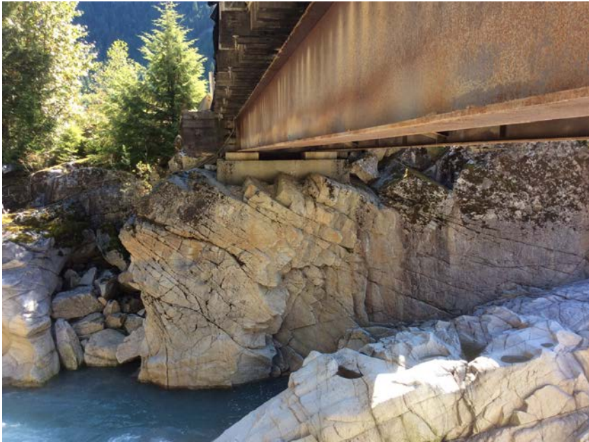
Right Bank Abutment when facing downstream
